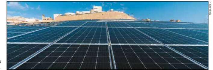
Self-sufficient The SESAME light source is the first accelerator infrastructure to be powered by renewable energy, but not all facilities have that option.
